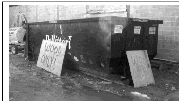
Figure 9. Findorff workers created these spray-painted plywood signs to label dumpsters after they were moved around to re-open Mifflin Street. May 2003.
